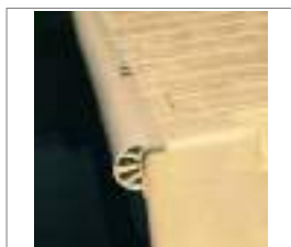
Dock edging including fixings
